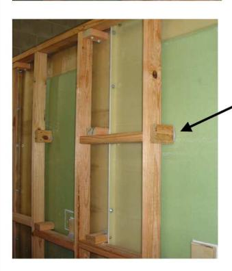
FIX STUDS TO BATHROOM WALL PANELS BETWEEN FLANGES LIKE THIS.
